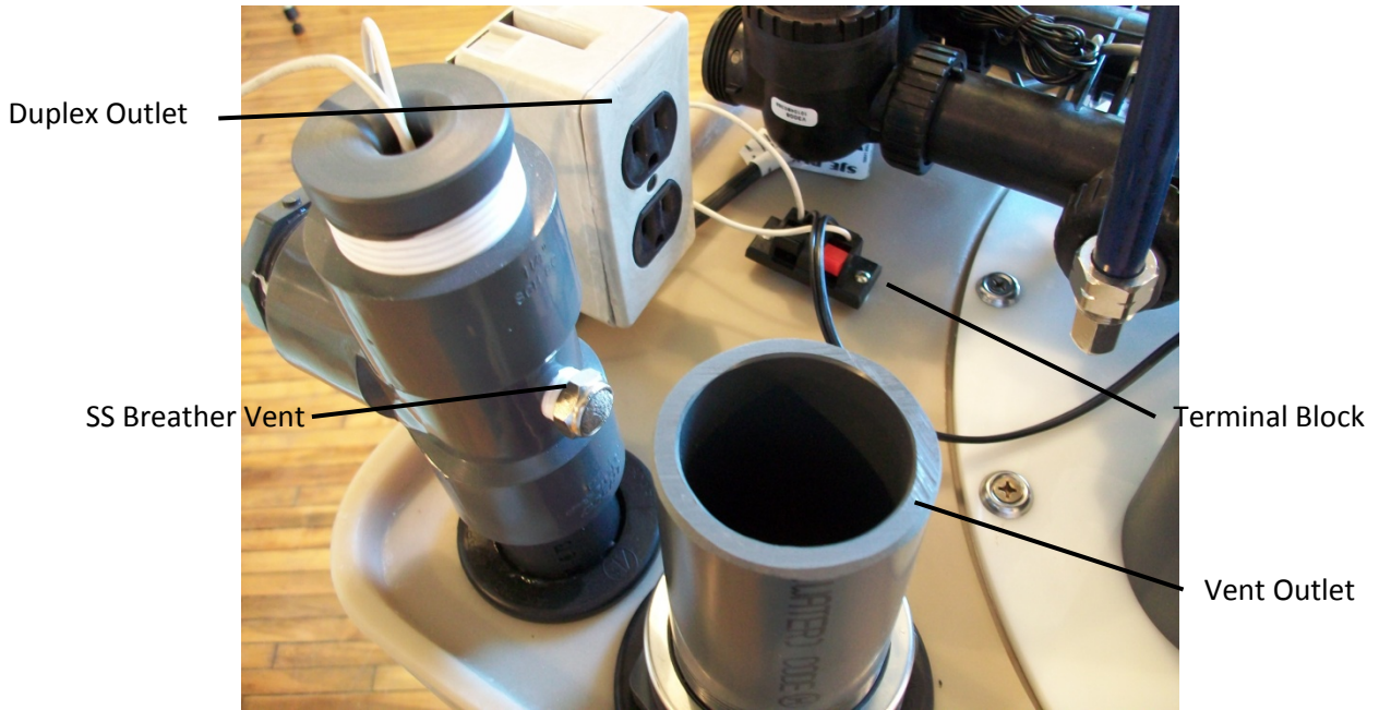
Figure 10 – Terminal Block and Overflow
